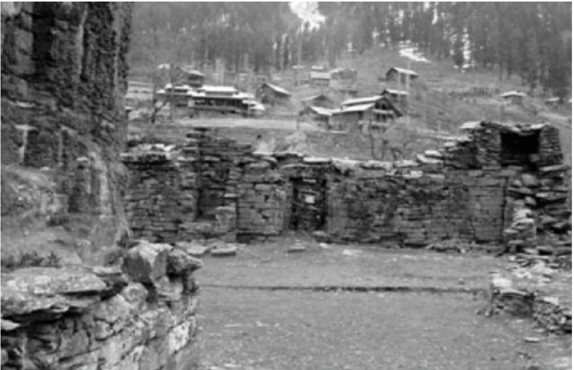
Inside of Sharda Temple complex : This photo was taken on 12th April 2005. Photo Courtesy : Hanif Gharib
